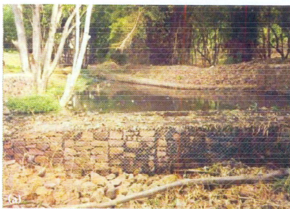
Fig. 1: Restoration and Mitigation activities for sustainable development of wetlands (a) Gabian structure to control flow of solid waste (b) Construction of Special Bank
