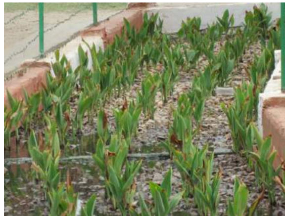
Figure 17.10 Treatment unit planted with Canna indica .
