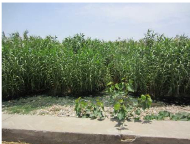
Figure 10.4 HSSF-CW (second step in tertiary treatment).
