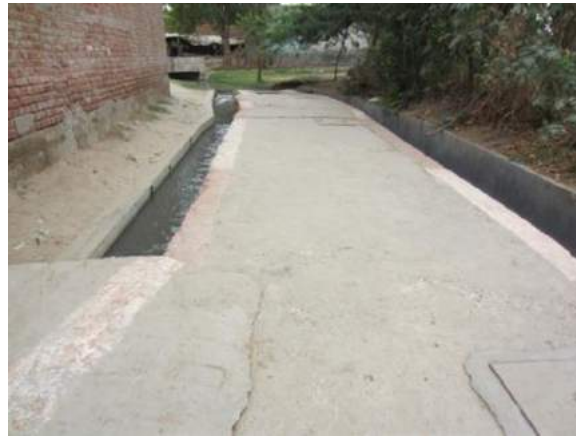
Figure 17.12 Primary treatment unit (baffled septic tank).
